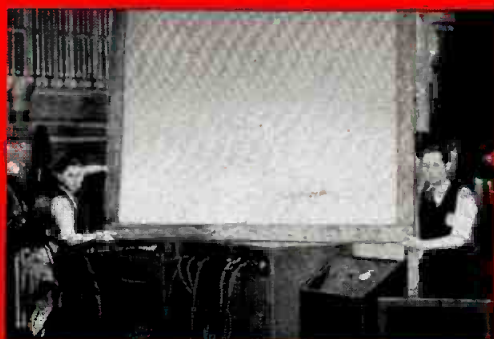
First Theatre Television. In May, 1930, Dr. Alexanderson produced a picture 7 feet square on a screen in Proctor's Theater, Schenectady. Receiver used a light cell developed by Dr. August Koralus.
